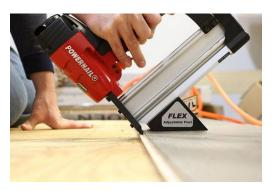
After laying the first board into the bead of glue, position the nailing machine so that the nail will enter the floor board at an angle between the upper lip of the tongue and the face of the floor(see photo right). We recommend an 18-gauge cleat (1-1/4"-1-1/2" length), nailing every 6 inches. The first
